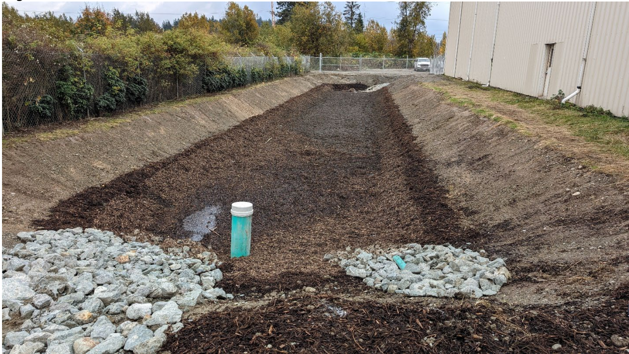
Photo 9. Bioretention Cell Before Vegetation
