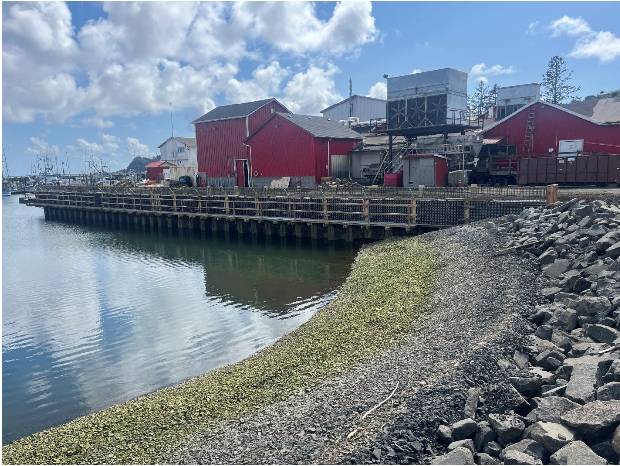
Photo 6. Active construction of Safe Coast Seafoods Bulkhead
